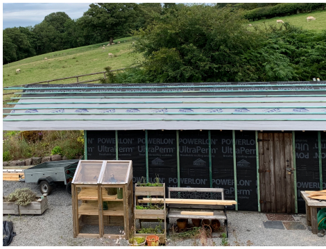
New Roof Ready For Slates
