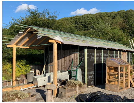
Roof Overhang Posts
