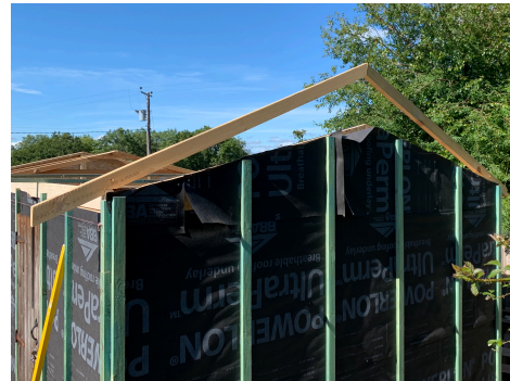
Removing Old Roof
