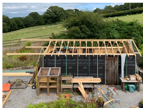
New Roof & Overhang
