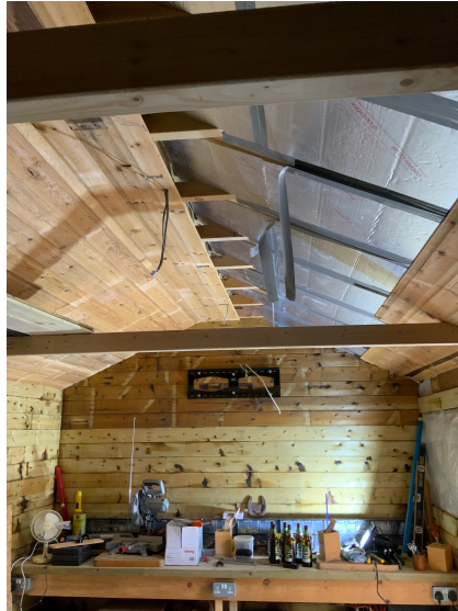
Roof insulation & cladding
