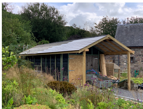
Slating The Roof
