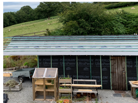
New Roof Ready For Slates
