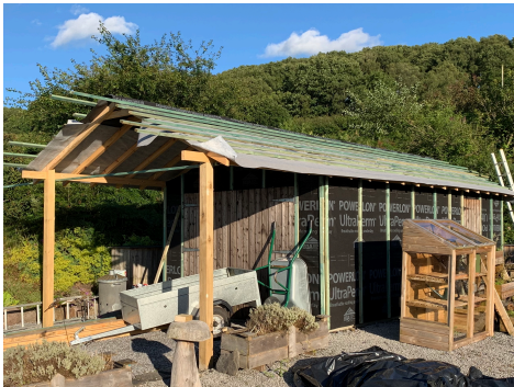
Roof Overhang Posts
